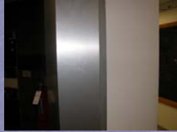
24 Inch thick walls
